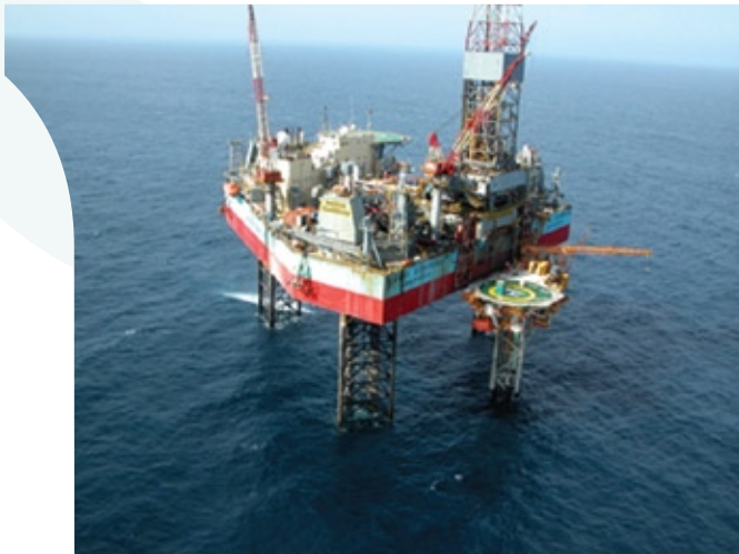
Woodside's Thylacine platform - Otways
